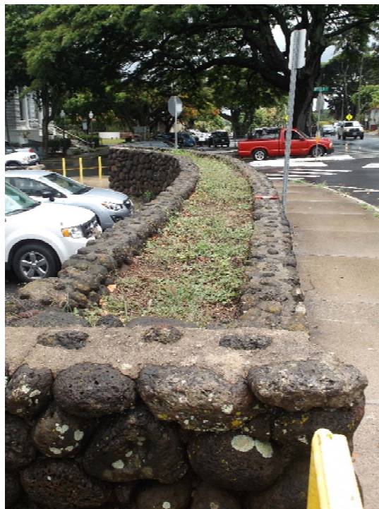
Figure 24. Portion of the western wall segment showing double wall construction, facing south.
