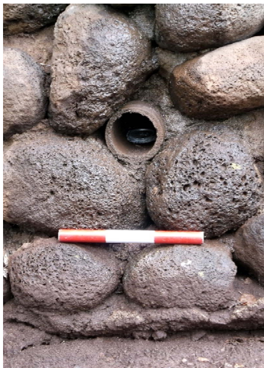
Figure 22. Portion of the east wall segment showing cement drainage pipe, facing west.
