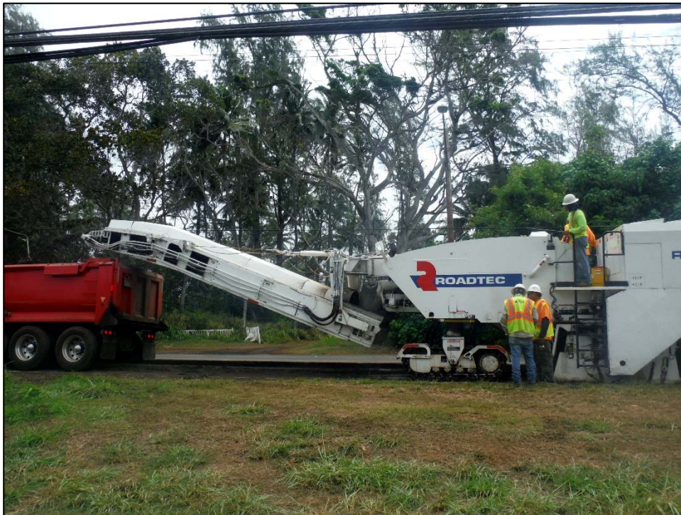
Figure 10. Excavation with coldplaner.
