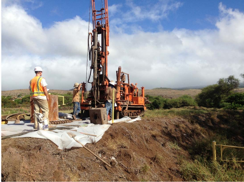
Figure 25. Boring at B-10, showing the drill rig atop the levee wall. View is to the northwest.
