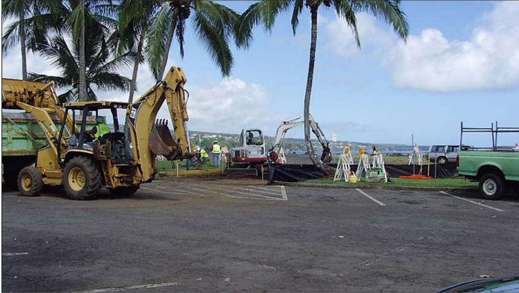
Figure 9. Example of equipment used on the construction site. A backhoe and mini excavator are shown.
