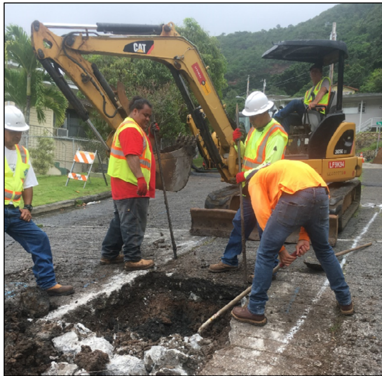
Figure 12. Excavation with a mini excavator and shovels.
