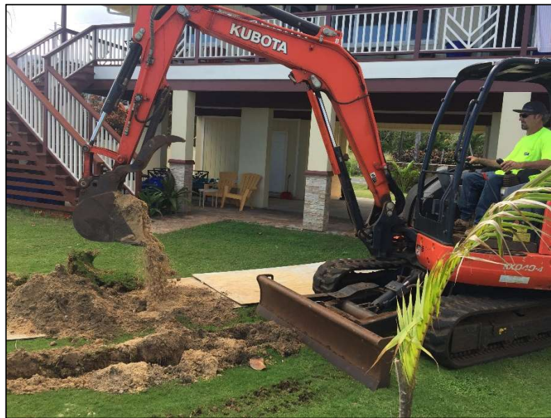
Figure 8. Excavation of trench with mini excavator. Orientation is to the south.
