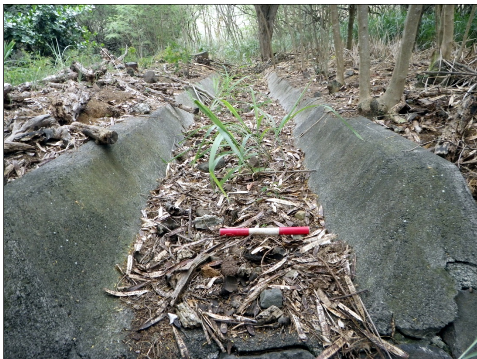
Figure 14. Site 50-80-15-7318 drainage ditch, facing northeast. The stone interior can be seen in the foreground beneath the concrete lining.
