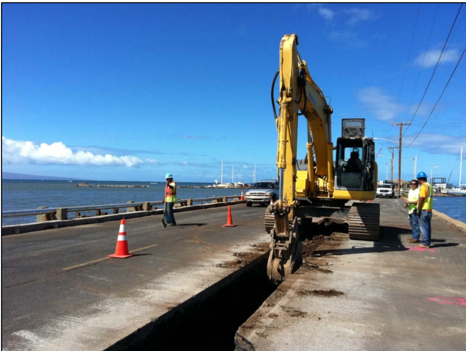
Figure 22. Trenching with the excavator.
