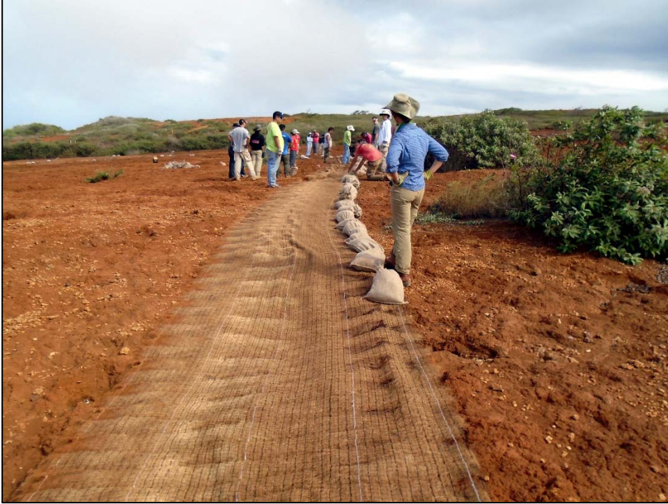
Figure 6. Volunteers extending the wattles at Site 704 to prevent artifacts from eroding downslope. View is to the east.
