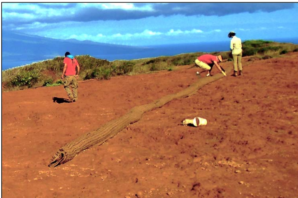
Figure 23. Construction of a wattle between Features 522A (right of wattle) and 522B (left of wattle). View is to the southeast.
