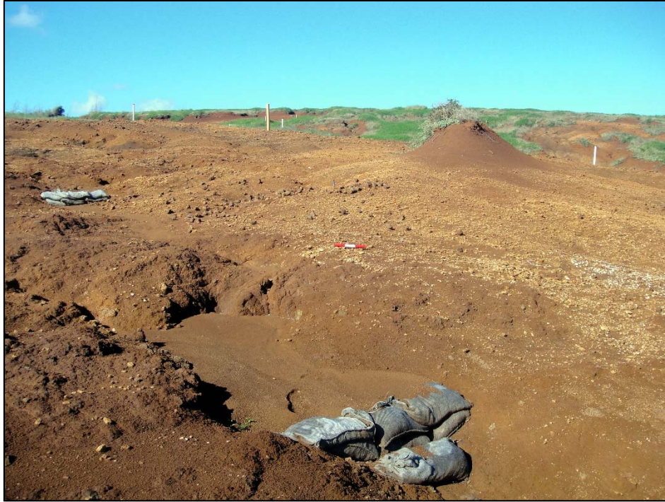
Figure 21. Site 520 erosion control measures implemented, facing west. Note the buildup of sediment on the upslope side of the barrier, indicating that erosion is being curbed.
