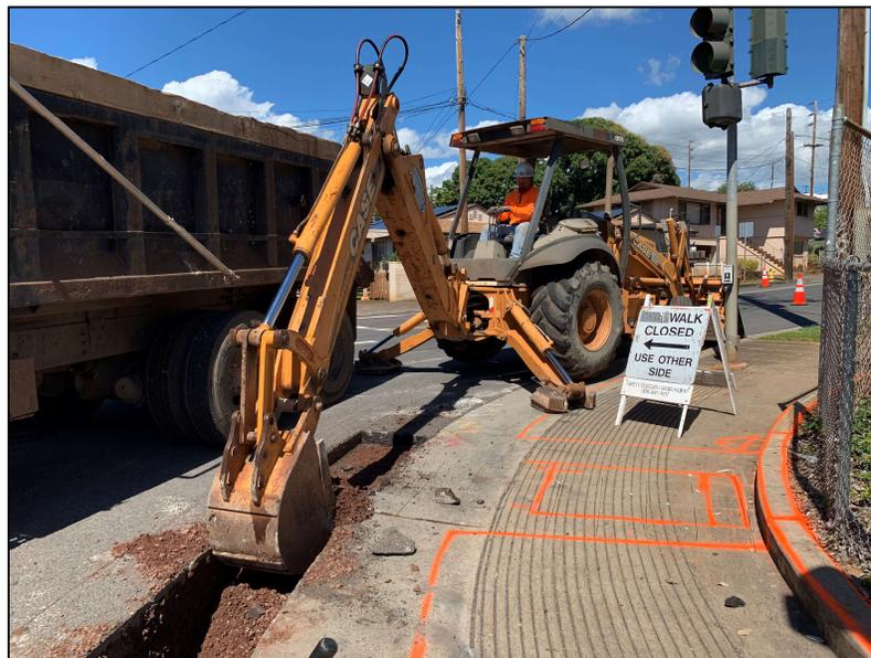
**Figure 10. Excavation with a backhoe.**
