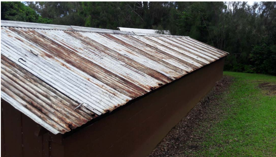
Makaha Cabins, rusted roof. Orientation is to the north.
