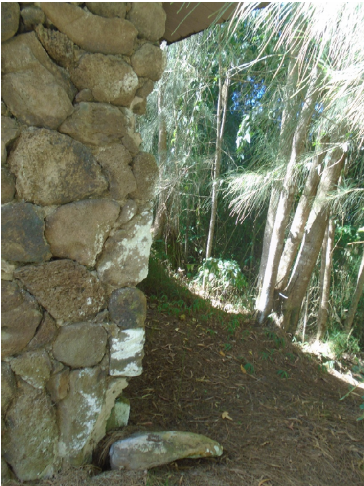
Stones falling and missing from north corner of the building. Orientation is to the west.
