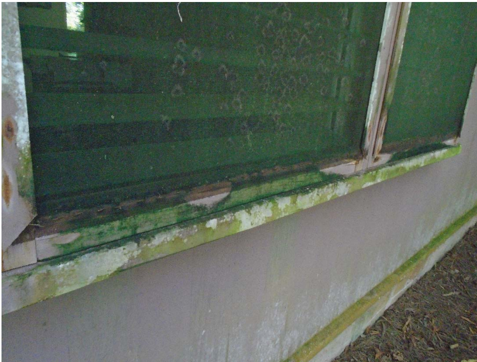
Rotted window frame with boards missing. Orientation is to the east.
