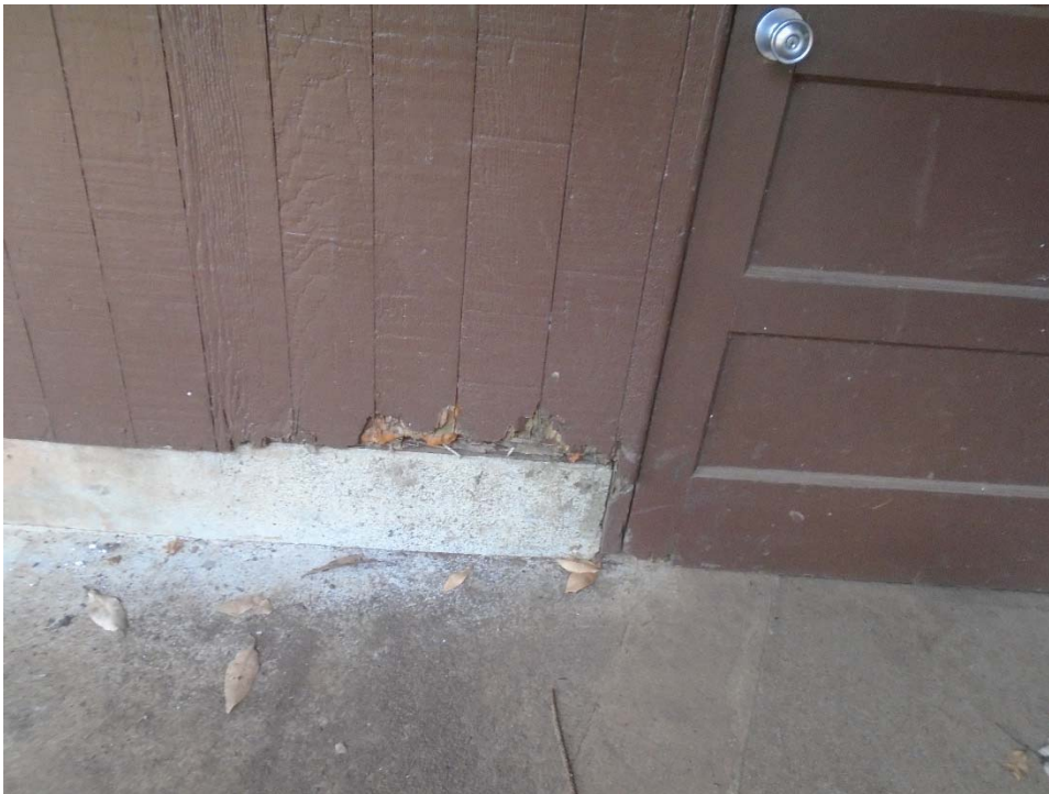
Wood rot near door at front of building. Orientation is to the east.
