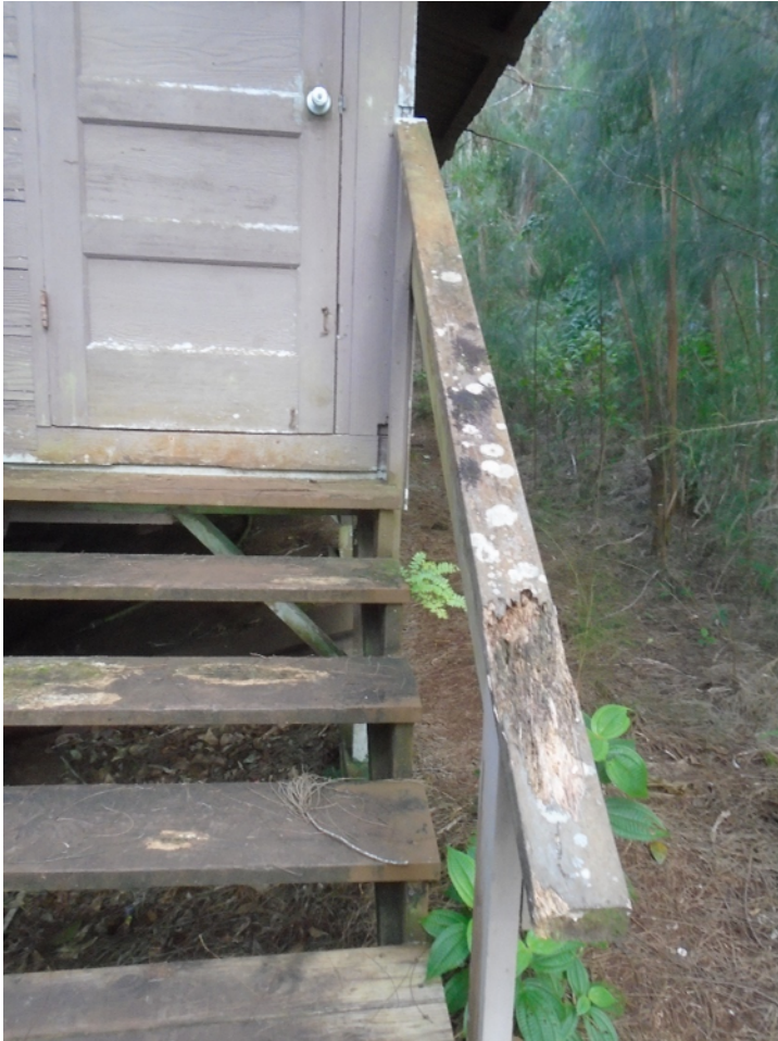
Wood rot on stair railing. Orientation is to the northeast.
