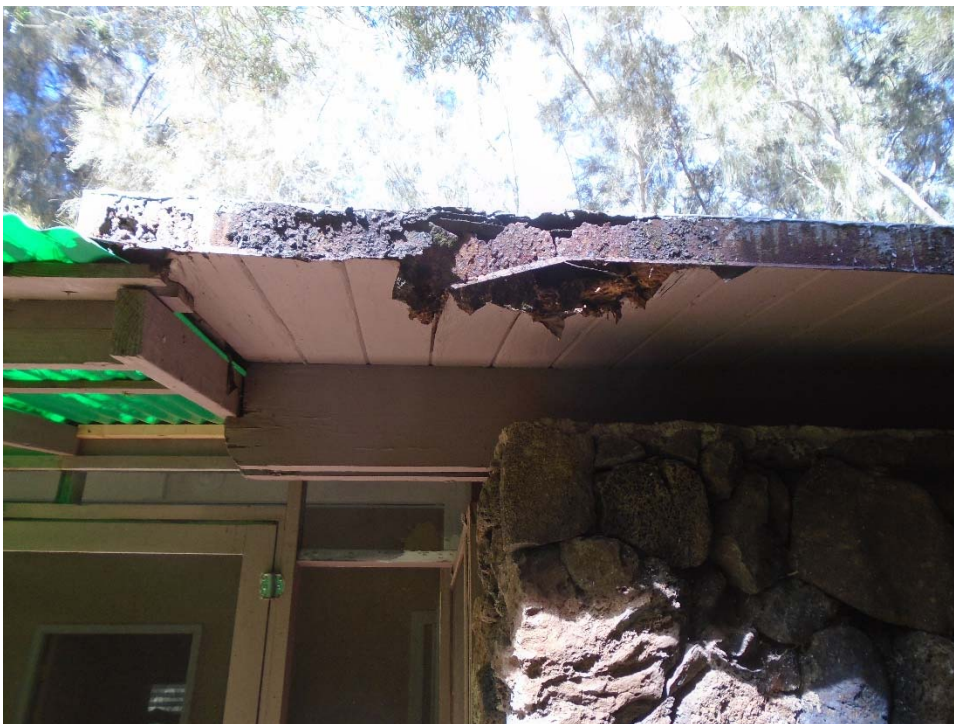
Wood rot and metal siding rust. Orientation is to the west.
