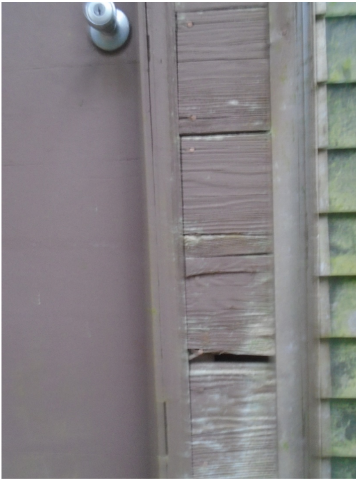
Wood rot near back door. Orientation is to the southwest.
